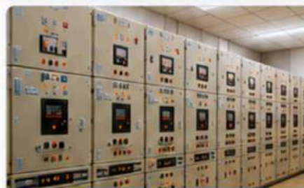
HT / LT SWITCHGEAR INSTALLATION
