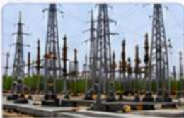
Switchgear & Switchyard Erection
