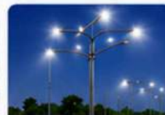
Yard Light Erection
