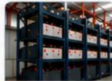
Battery Bank Installation
