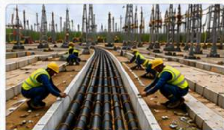
CABLE LAYING & CABLE TRAY ERECTION
