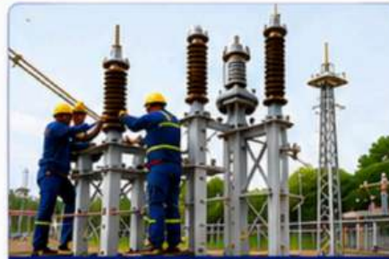
SWITCHYARD ERECTION
