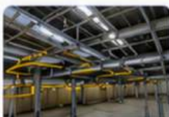
Cable Tray Erection
