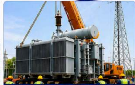
POWER TRANSFORMER INSTALLATION
