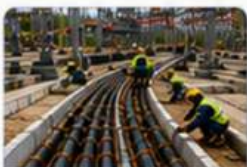
Cable Laying & Termination
